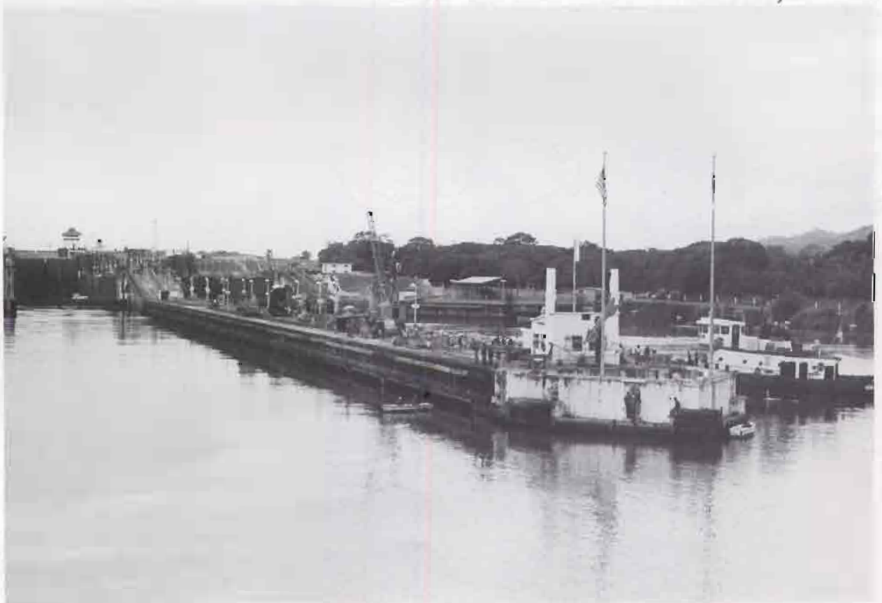
Entrance to the Mira Flores Locks on the Atlantic side
