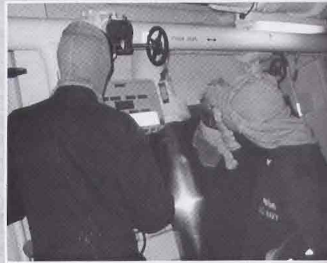
EM2 Malone, EM3 Smith, and EM3 Estrada electrically isolate a space.
