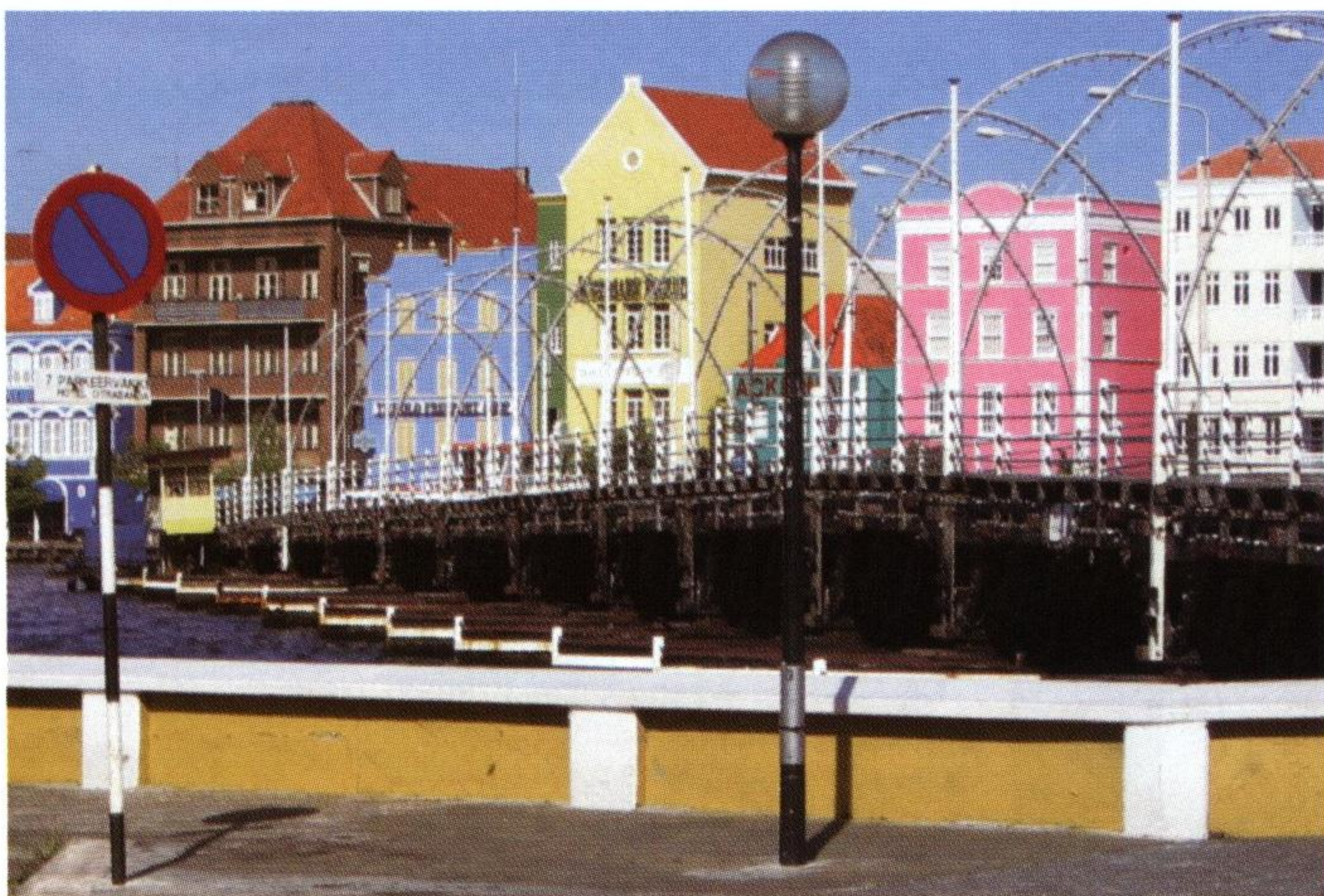
The bridge in the foreground floats on pontoons. When a ship is coming by, the bridge swings open.
